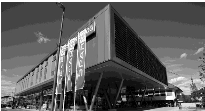
Figure 10: The new commercial building in Zalog in oversized format (photo: Domen Grögl).
