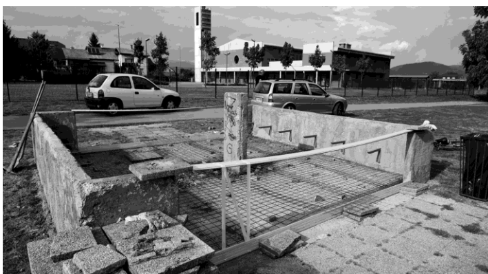
Figure 4: Action planning – renovation of the water well on the playground in Zalog as part of urban acupuncture process (photo: Domen Grögl).
