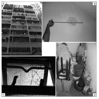
**Figure 2:** Physical and hygienic conditions of building B; a) front building elevation; b) concrete spalling on stairwell wall; c) cracked glazing of stairwell window; d) items in the stairwell (photo: Yung Yau).
