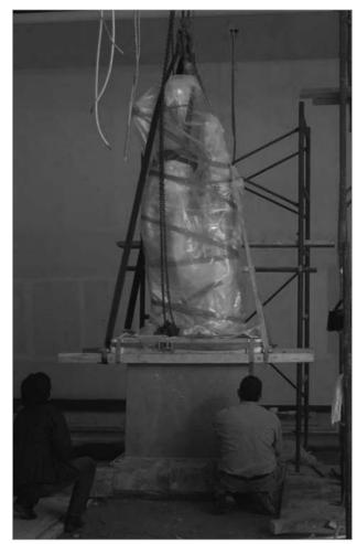
Figure 3: Placing the statue onto seismic isolation (source: Koumousis, 2007).
