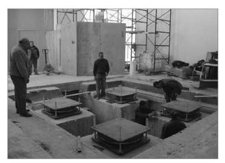
**Figure 2:** Installation of seismic isolation for the statue of Hermes at the Olympia museum (source: Koumousis, 2007).
